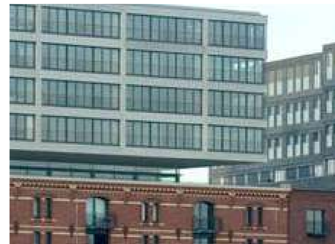
overgang dmv insnoering
