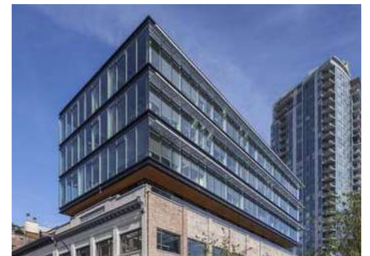
overgang dmv insnoering
